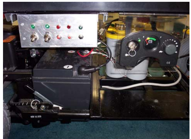
Figure 5.B - View of Circuit Box Mounted
